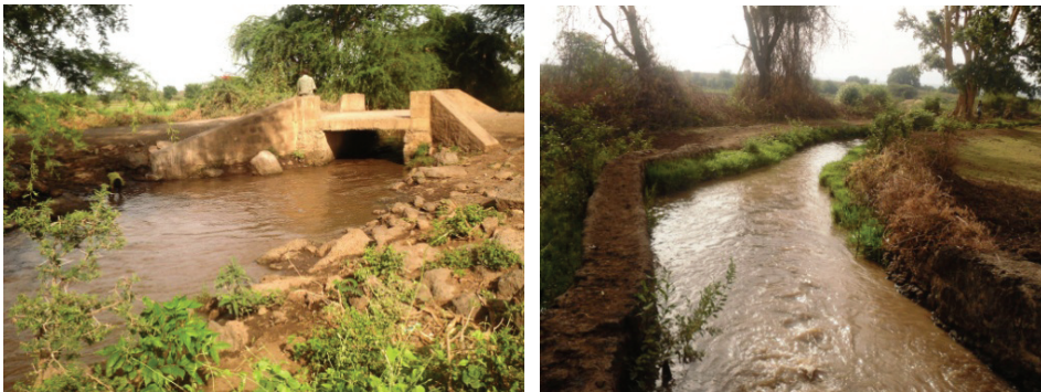
Figure 9.2. Flow at the head of an irrigation block at Golgota Scheme (lacks adequate farm structures for delivery to farthest outlets)
