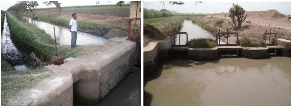
Figure 6.7. Low stage in a parent canal behind offtakes in the middle reach
