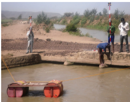
a. Measuring details of structures
