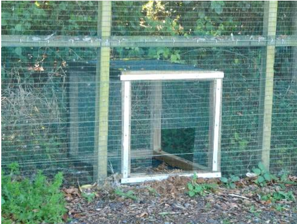
Figure 5. A cage as installed at the fence. The temporary mesh cover has been removed and the simulated 'flood-scour' breach is open.
