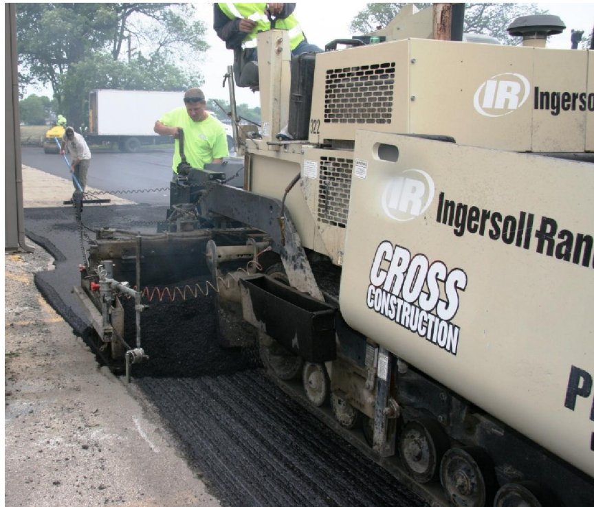
Figure 7-1 Asphalt mixture laid down by a paver.
