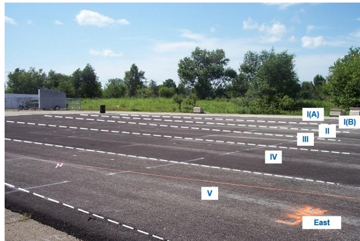
Figure 3-4 Existing test site (test site A) (40).
