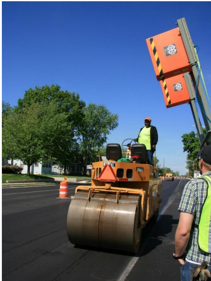
Figure 7-8 GPR antennas raised up to avoid disruption to roller.
