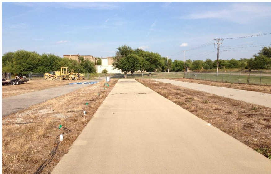
Figure 3-5 Existing pavement before construction of test site B.
