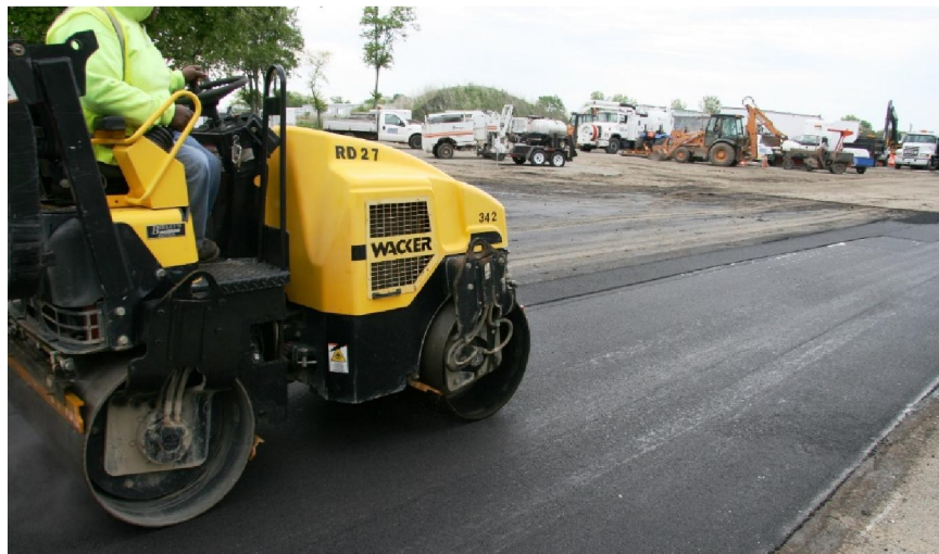
Figure 7-2 A vibratory steel roller on the asphalt pavement.
