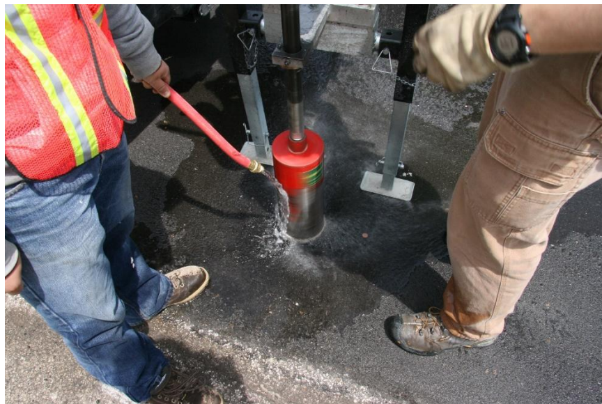
Figure 7-4 Core extraction at the location of GPR measurement.
