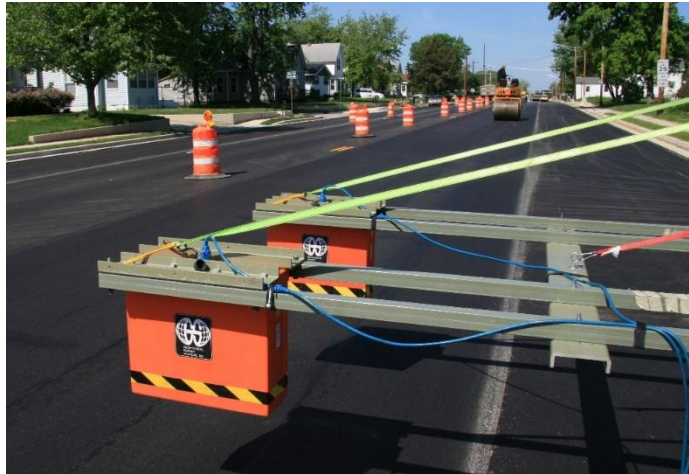
Figure 7-7 GPR data collection during compaction.
