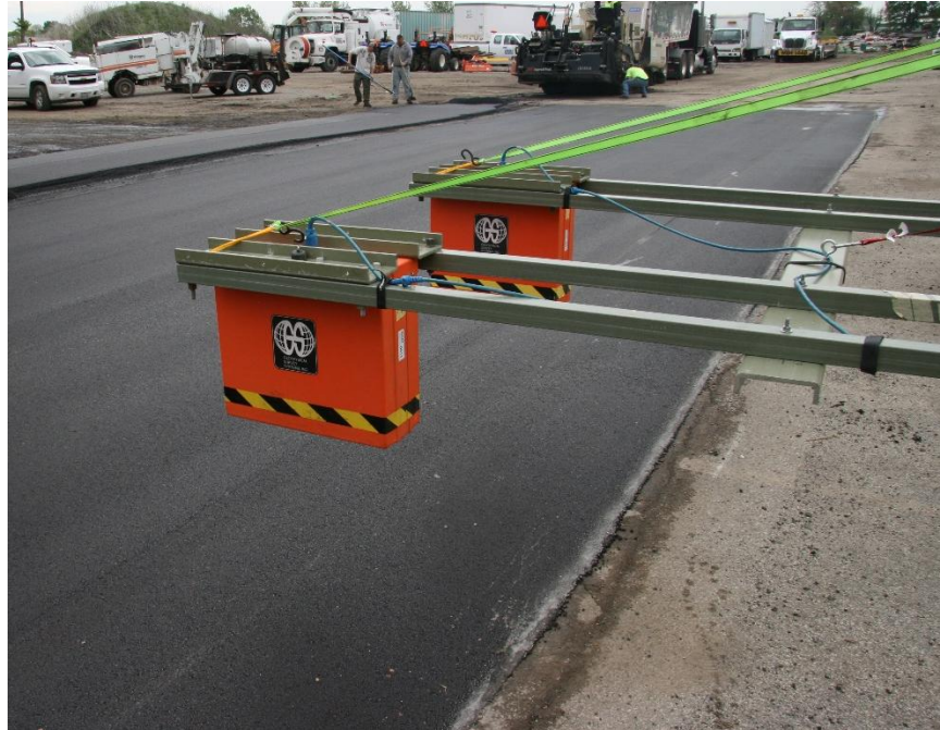
Figure 7-3 GPR data collection on dry pavement.
