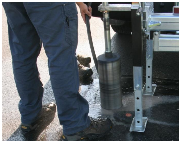
Figure 2-1 Core extraction from asphalt pavement.
