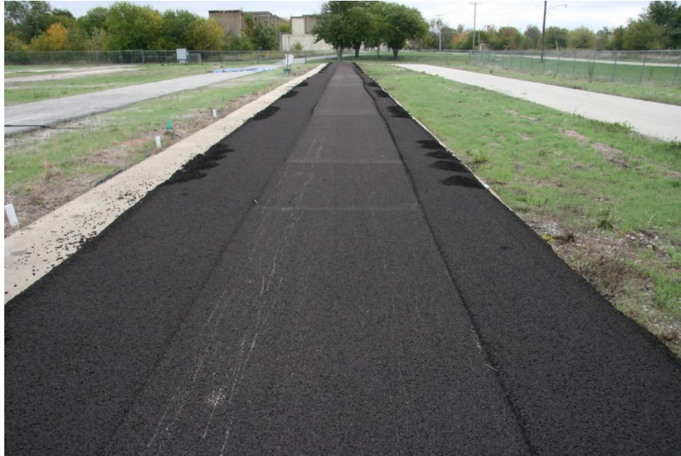
Figure 3-8 Test site B after construction.
