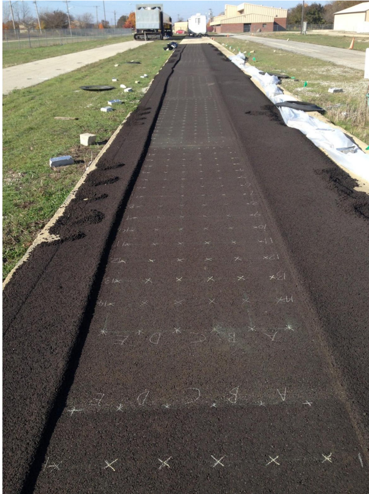
Figure 3-10 Grid system for location referencing on test site B.
