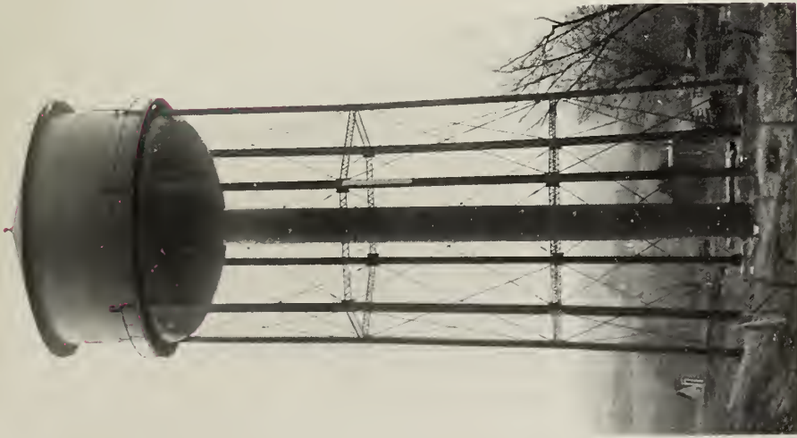
Patented Elliptical Bottom Tank with Parabolic Posts
