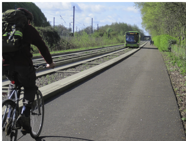
Fig. 1. The Cambridgeshire guided busway
