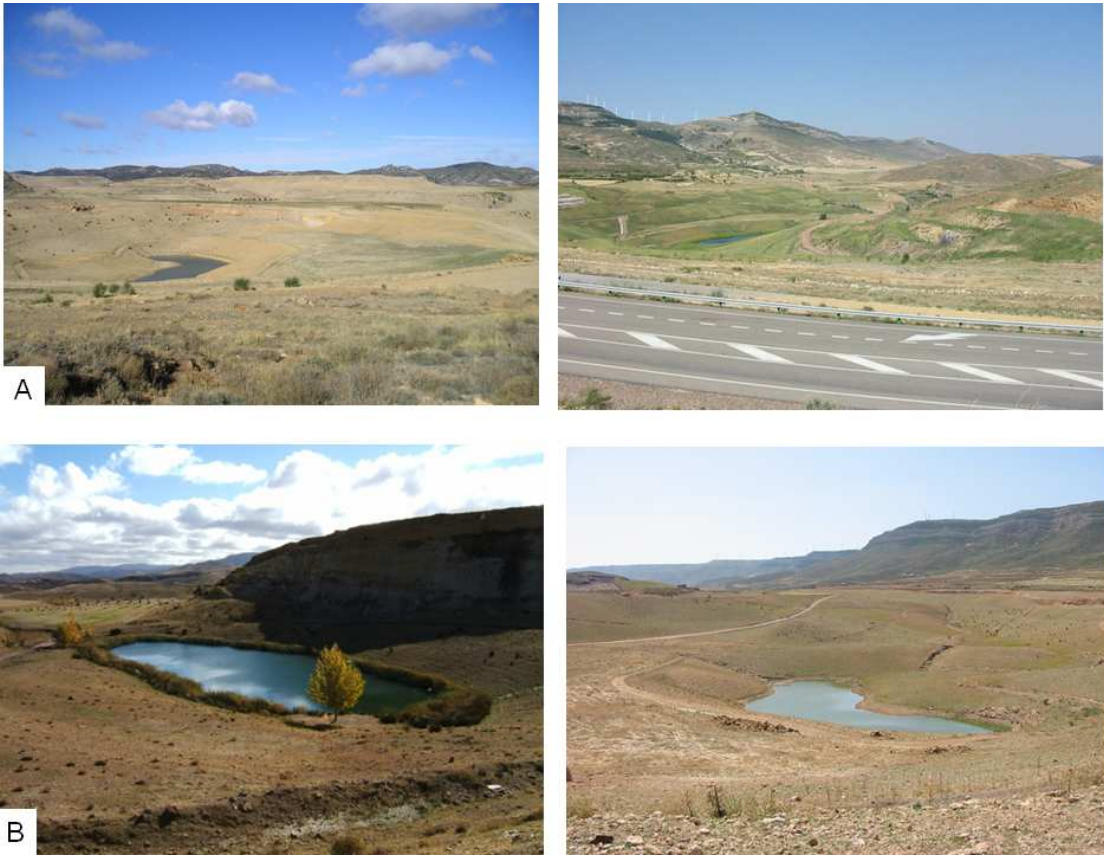
Fig. 11. Third generation of restoration (Utrillas) based on the understanding of the hydrological basin as a restoration unit. Reservoir works as a firebreaks line avoiding sediment emission to the natural watercourse and reducing peak flow.
