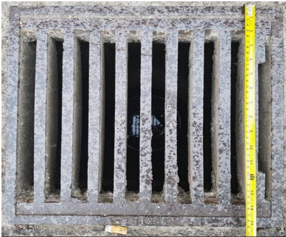
Figure 13 Dimensions of grate type inlets in Lomma town (42 cm X 40 cm).
