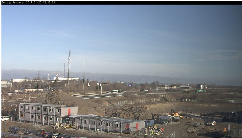
Figure 24: Sample frame of the Construction scene.
