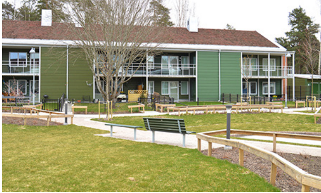
Fig. 21. Defined courtyard in Vivalla.
