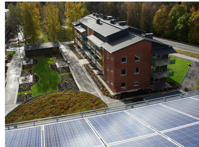
Fig. 22. Roof solar panels and renovated courtyard in Ålidhem.
