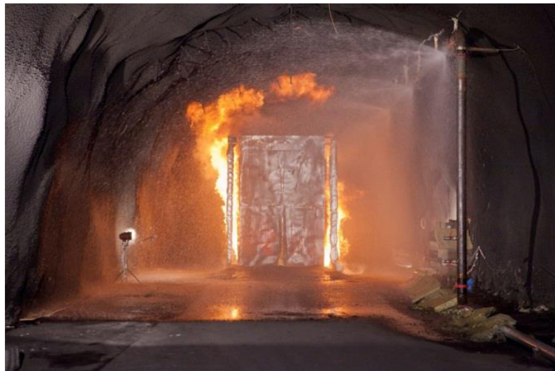
Figure 1 FFFS after activation of the system. With permission of SP [2]
