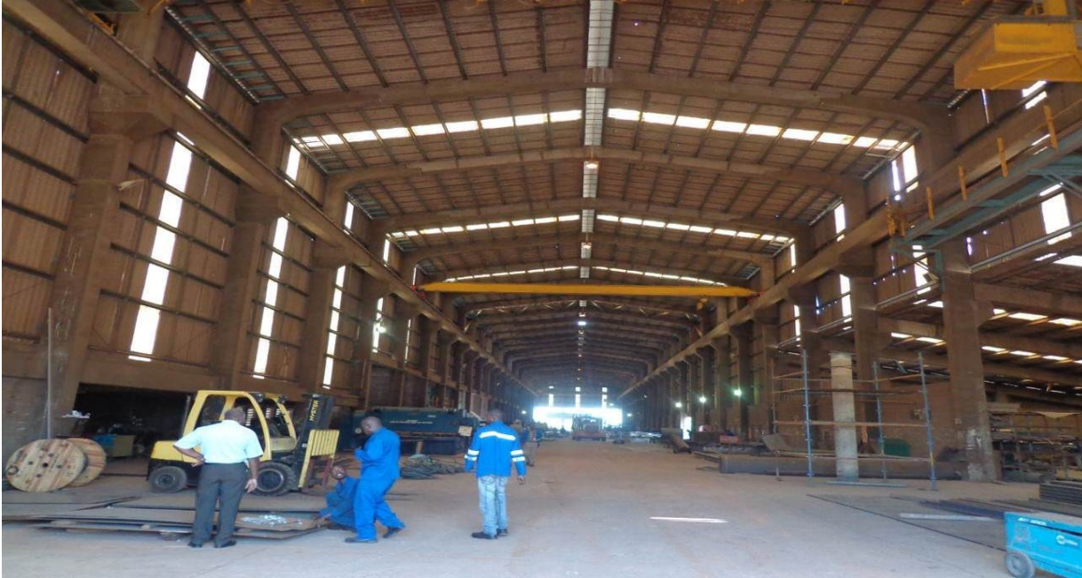
Figure 7: Example of Firms' Plant/Workshop
