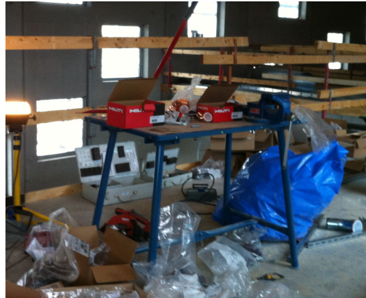
Figure 6.8 Workbench, construction site 4
