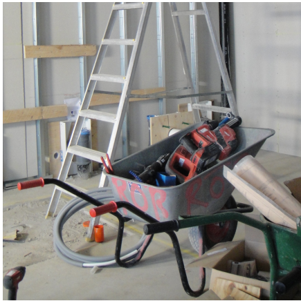
Figure 6.7 Wheelbarrow as workbench, construction site 3
