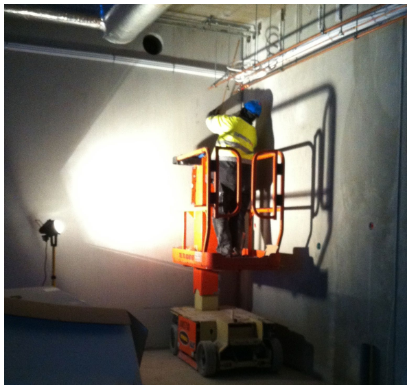
Figure 6.10 P&H installer covers the light source
