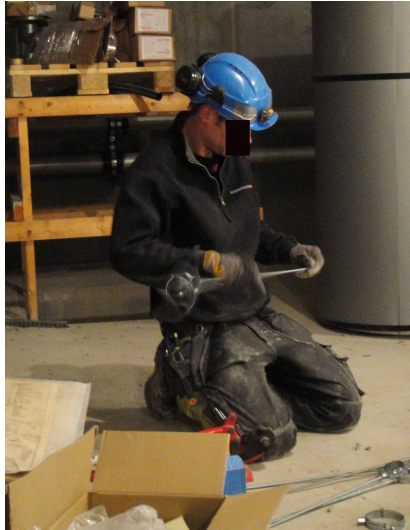
Figure 6.9 Preassembly performed on the floor by an P&H installer
