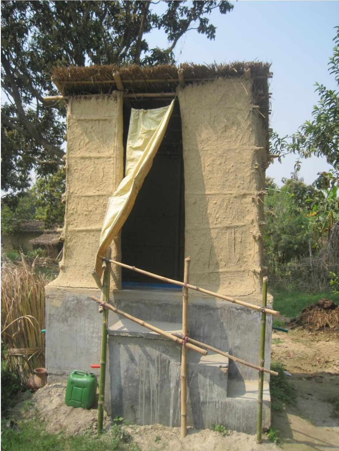
Figure 6: A completed UDDT. The substructure includes the concrete chamber and the stairs. The superstructure refers to everything on top of the concrete. The household have made the super structure out of grass, bamboo and mud. They have also chosen to erect a hand rail to help elderly members (Photo taken by Myers, 2013)
