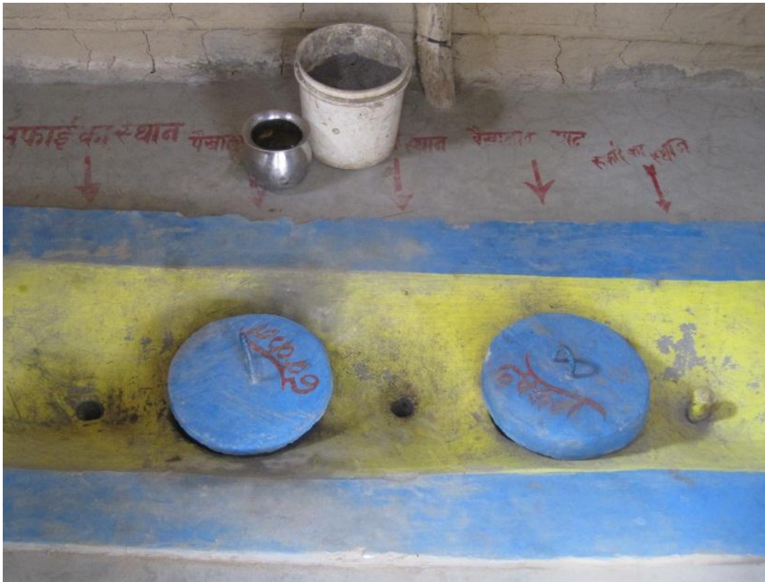
Figure 5: A picture of the top of the sub-structure. What each hole is for is written in Hindi. The chamber on the left of the picture is currently in use (Photo taken by Myers, 2013)
