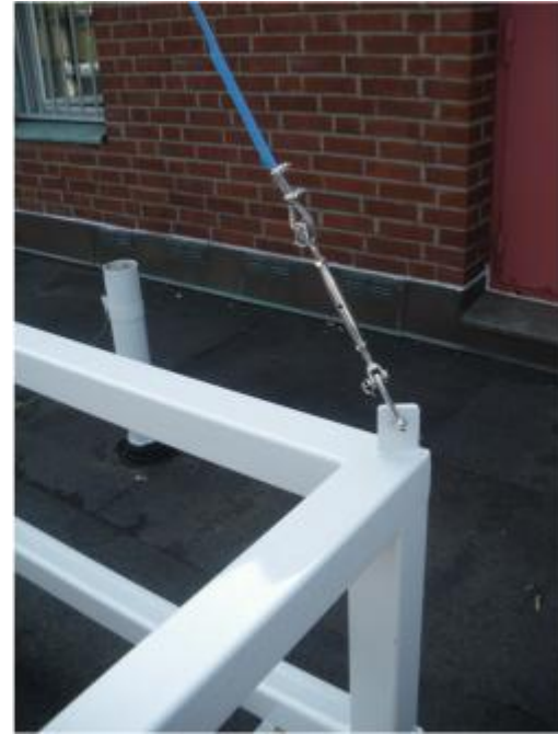
Picture 4: safety wires connecting the mast to the structure
