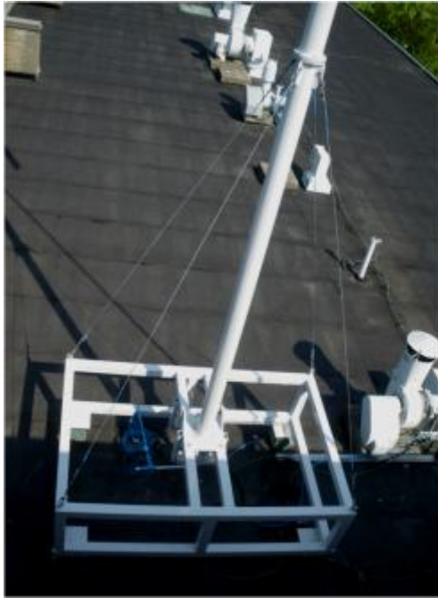
Picture 4: safety wires connecting the mast to the structure
