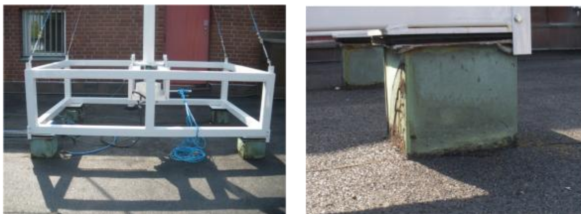
Picture 2: Base of the structure and plinths supporting it
