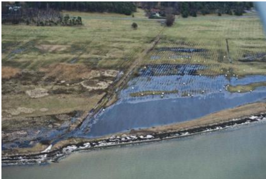
Figure 55. Photo (Gustavsson 2011) taken after the storm 2011-11-27, section including profile 9. Seaweed has washed up 15 m.
