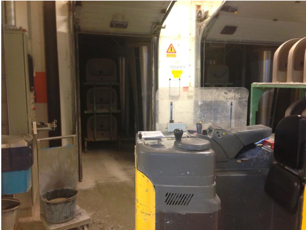
Figure 15 - South 1 dryer, with pieces on racks inside and the production line forklift in front
