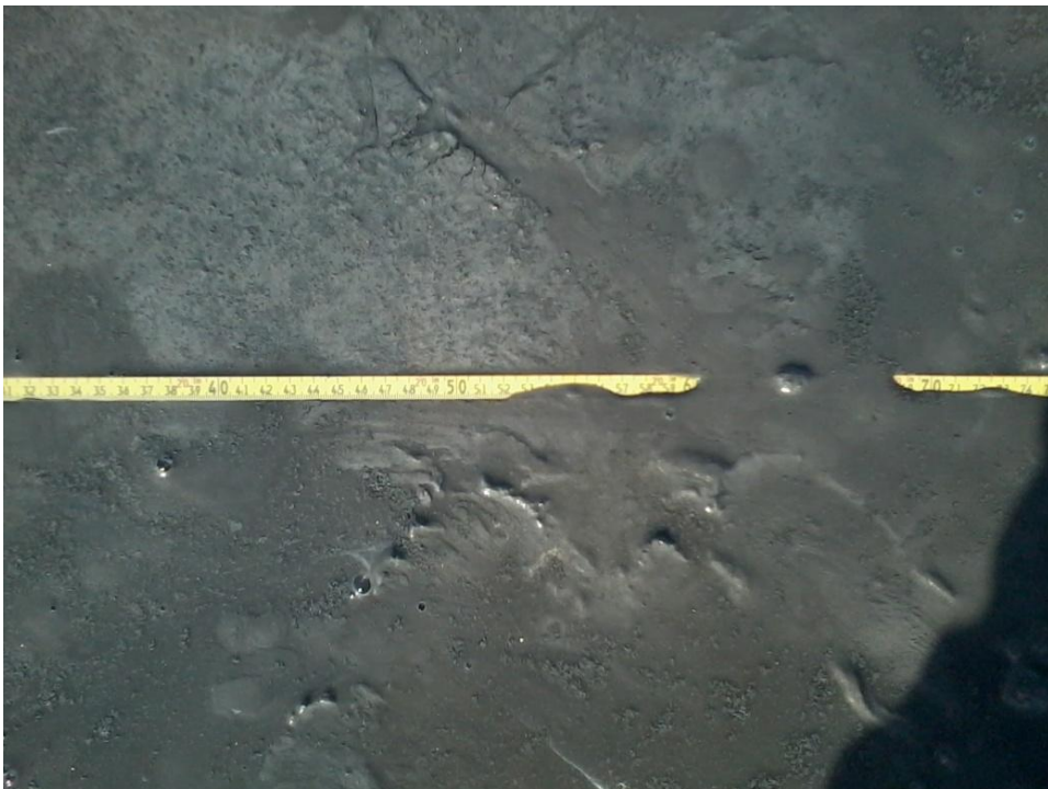
Figure 5-15: 120 m from dam wall 2013-09.
