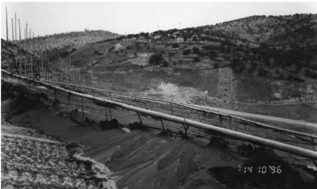
Figure 2-7: Spray bars during deposition (Blight, 2010 p. 314).
