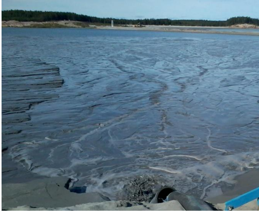
Figure 3-2: Delta created by flow from spigots at Garpenberg tailings dam C, 2013-09-03.
