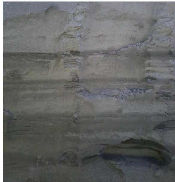
Figure 5-6: Layering in trial pit at dam A 2013-09.
