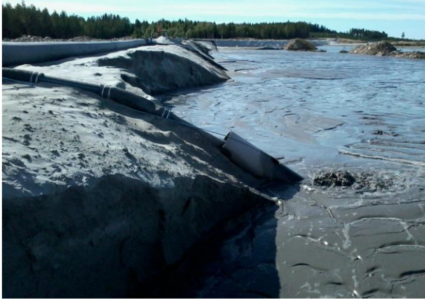
Figure 2-6: A spigot at the Garpenberg tailings dam 2013-09-03.
