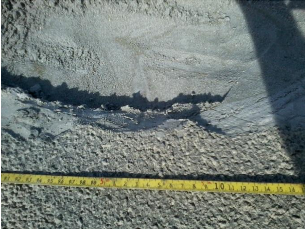
Figure 5-8: 5 m from dam wall 2013-09.
