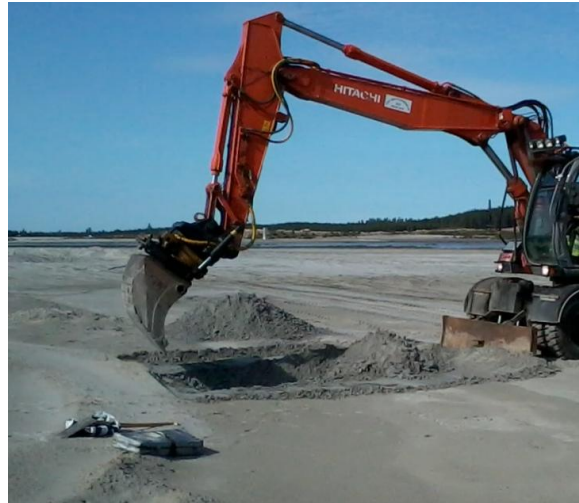
Figure 5-5: On-going excavation of a trial pit in dam A 2013-09.
