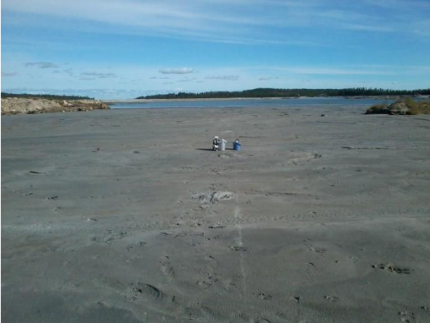
Figure 5-19: Beach at dam D section 0+850, 2013-09.
