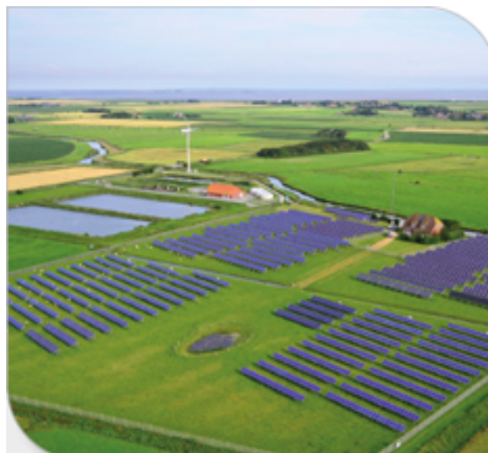
Figure 2.13: Picture of the E.ON hybrid power plant.
