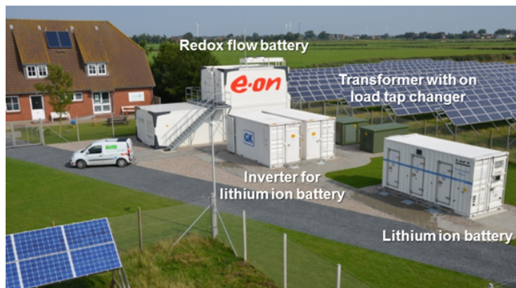
Figure 2.14: Storage system of Pellworm.
