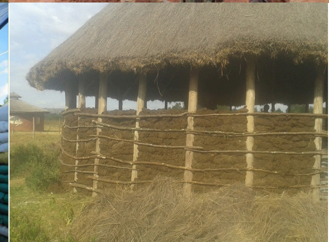
Picture 5 from top left: Biogas digester in Maili Saba demonstration garden, 6) Solar cooker (made from a carton box and silver foil), 7) solar panels, 8) manually making bricks, 9) building earth-bag-house, 10) kitchen house made of wood, mud and straw.
