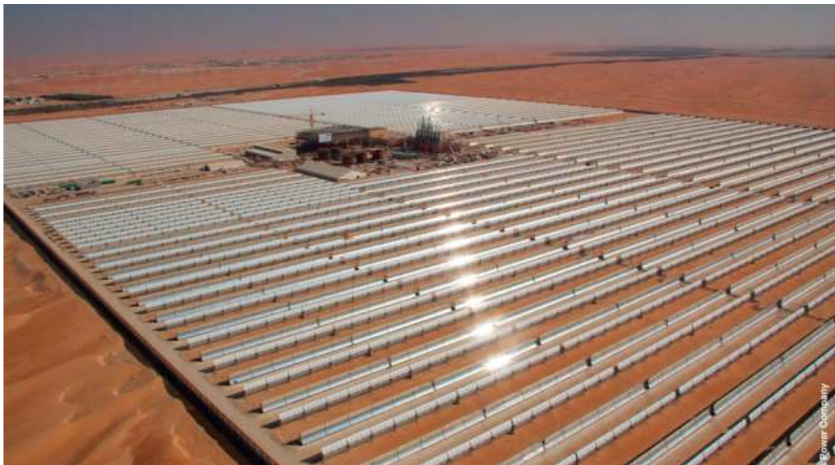
Figure 6: Construction site of NOOR 1 in Ouarzazate. Source: http://www.evwind.es/2014/10/20/first-concentrated-solar-power-csp-plant-in-morocco-solar-energy-project-to-open-in-2015/48190 The power of the sun: CDA of the Moroccan solar sector
