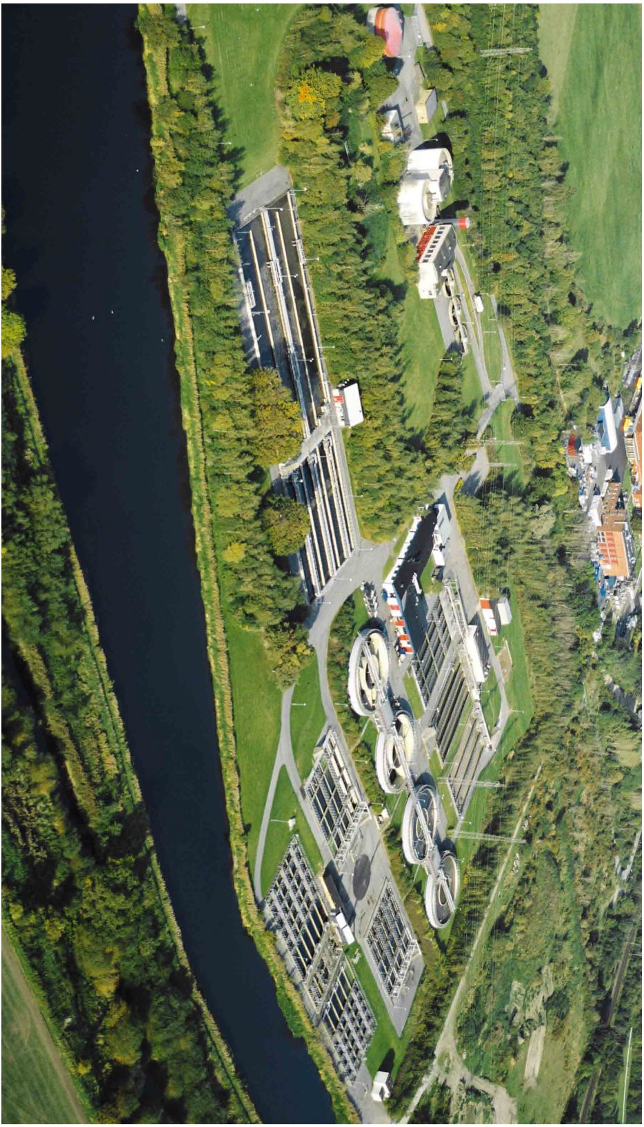
Figure 2.2: Aerial photo of Källby wastewater treatment plant (VA SYD, 2009).
