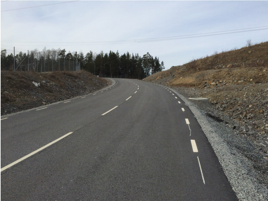
Figure 4.21 A photograph of the terrain. The ditch to the left is named Ditch 1 in figure 4.21, and the ditch to the right is Ditch 2. © Scania CV AB
