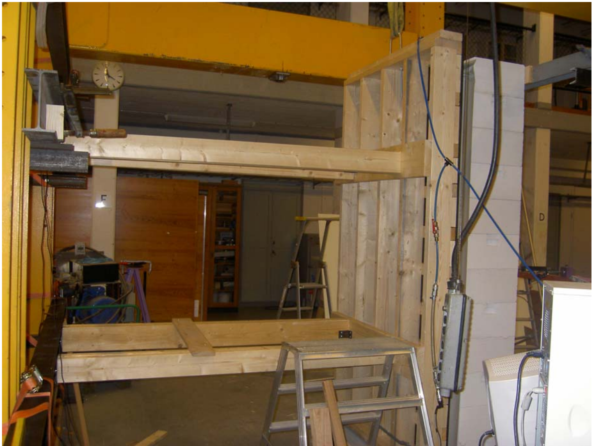
Figure 7. Struts attached to the resisting wall.
