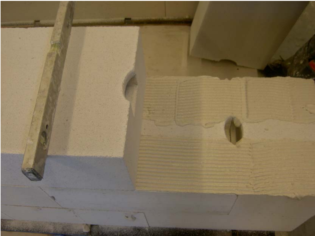
Figure 2. Mortar in strings of 150 millimetres with a half blocks displacement.
