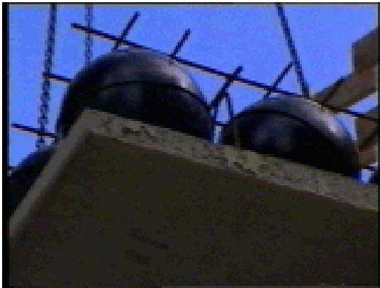
Figure 3.21 Bubble deck. [40]
