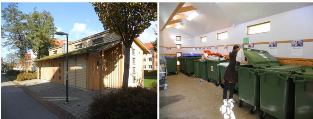
Figure 2. Exterior and Interior of the source-separation station in Augustenborg (Visual Image, 15 th , September, 2011)
