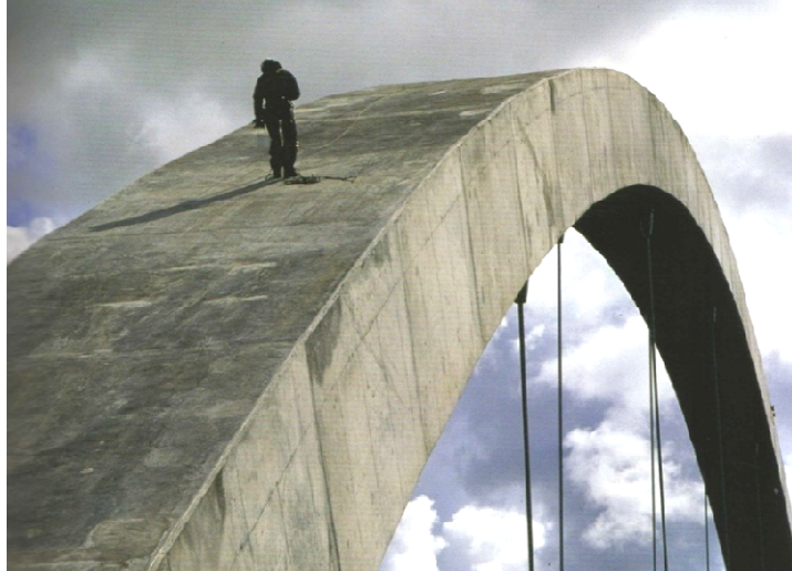
Figure 12 - Inspection of the concrete surfaces of the arch
