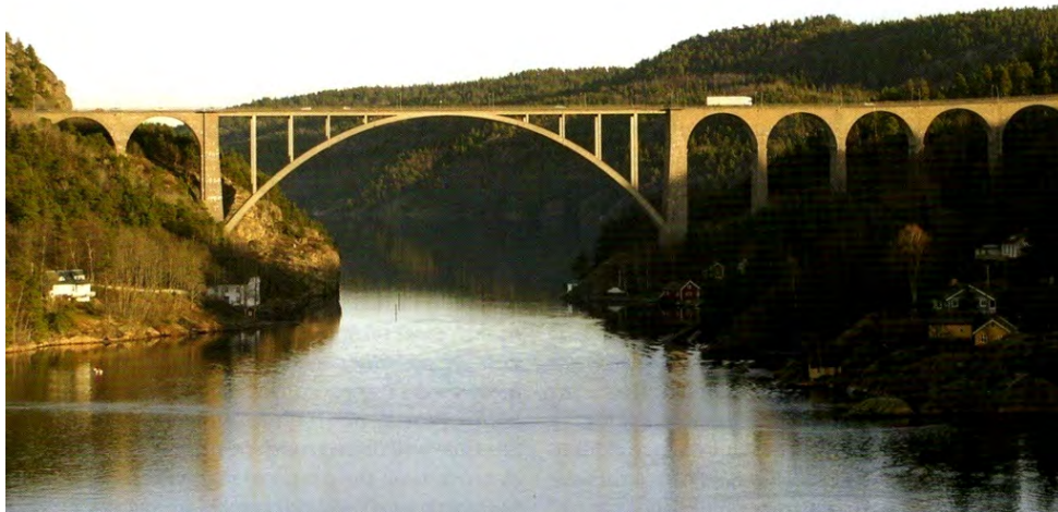
Figure 5 – The Old Svinesund Bridge made of reinforced concrete with approach vault bridges made of granite
