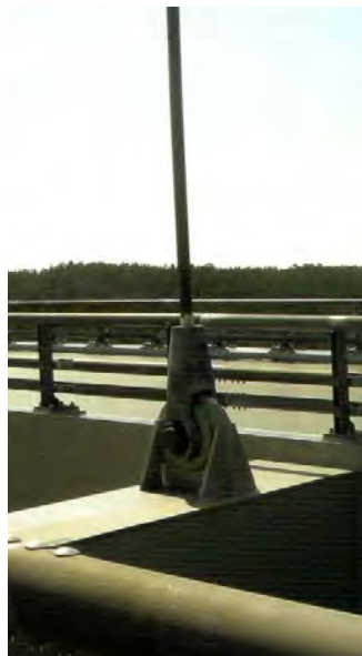
Figure 9 - Lower hanger attachment in cross girder
