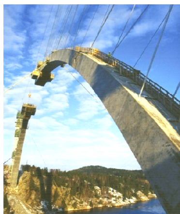
Figure 14 - Temporary staying the arch rib during the construction phase
