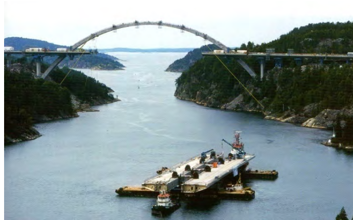
Figure 15 - Transport of the central sections of the superstructure by boat
