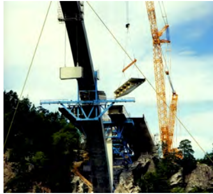
Figure 17 – Lifting sections of the superstructure using a mobile crane – Norwegian side
