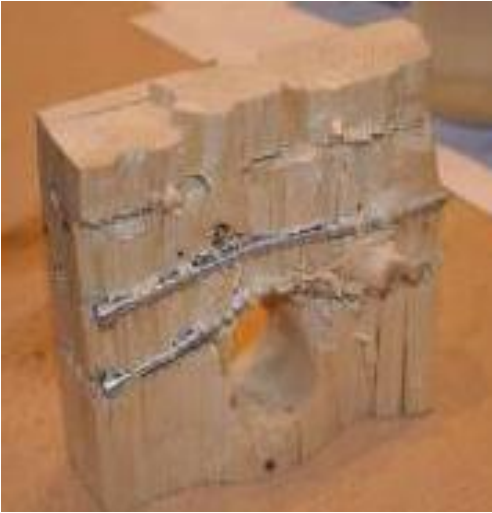
Figure 11 Typical failure mode for reinforced specimens. (Crocetti, Axelson, & Sartori, 2010)
