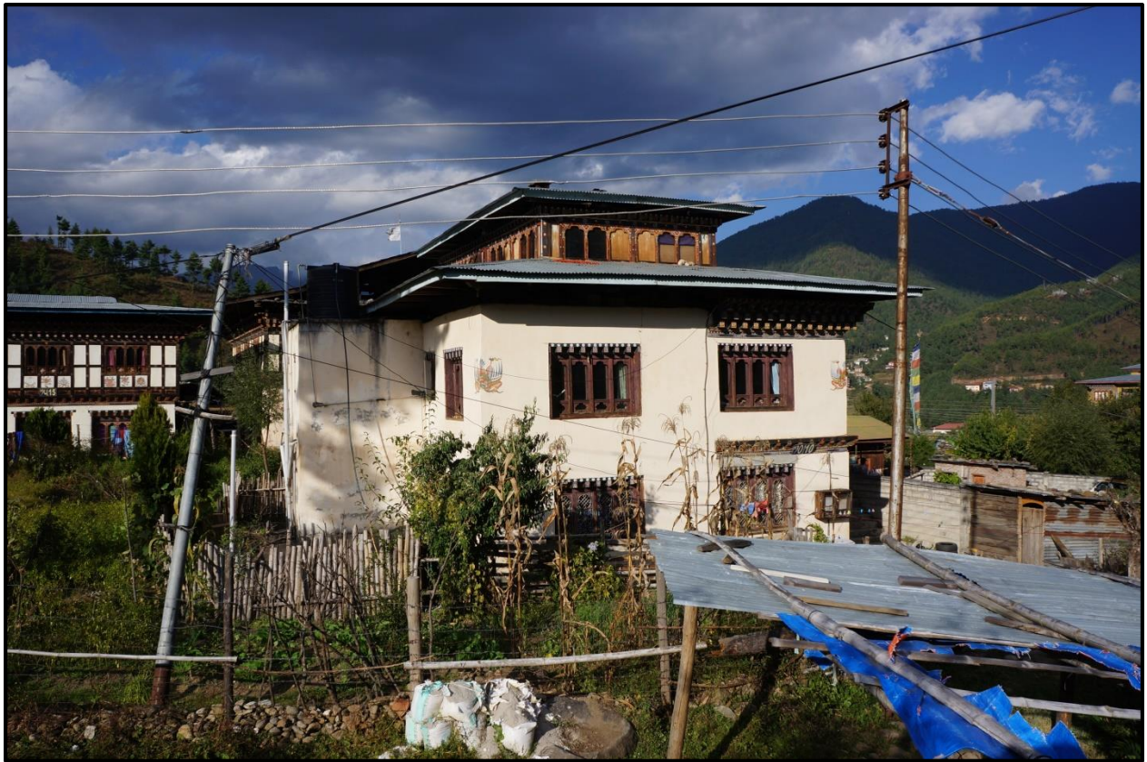
Figure 3.6.1.2: The wooden construction on top of this rural house is the Jamthog.
