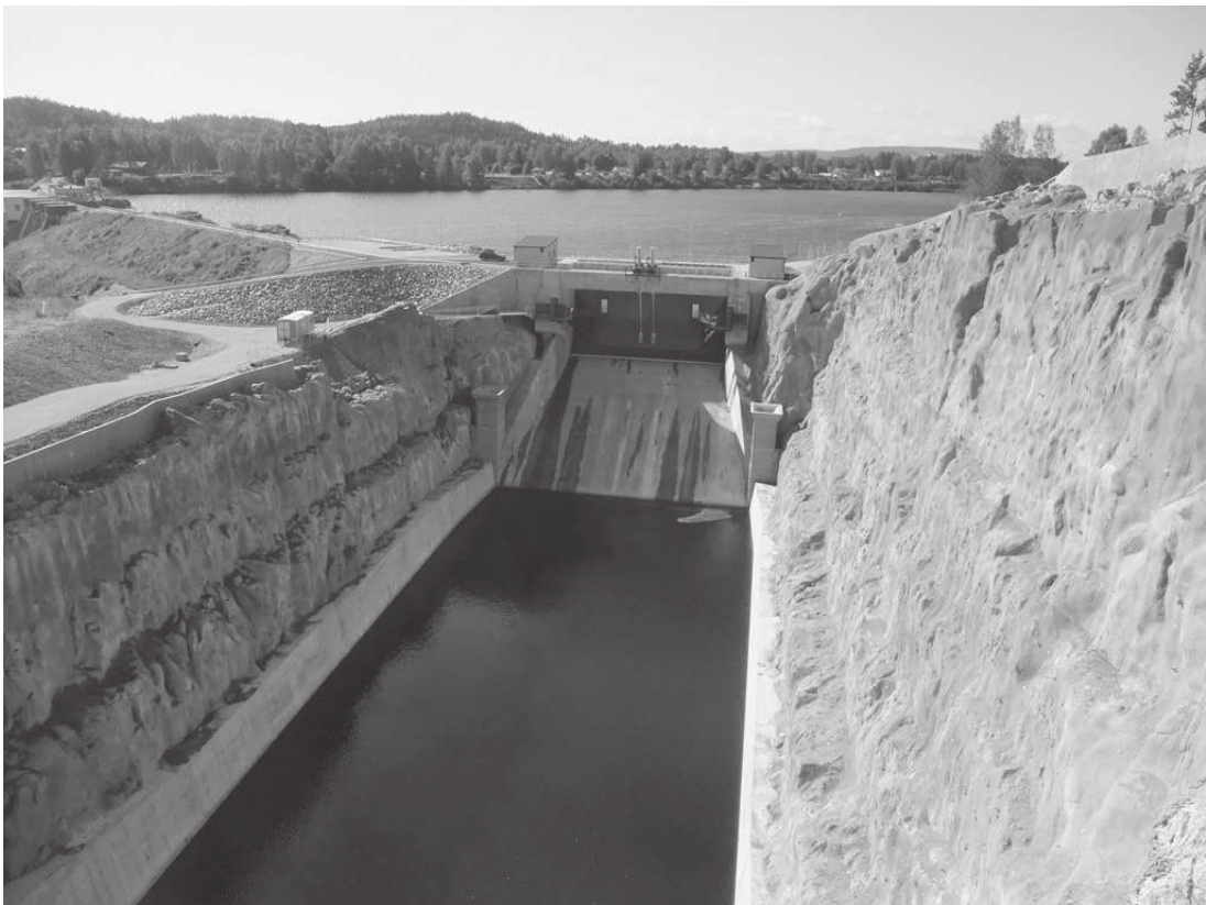
FIGURE 4.2: Spillway inlet viewed from downstream with aerator submerged
