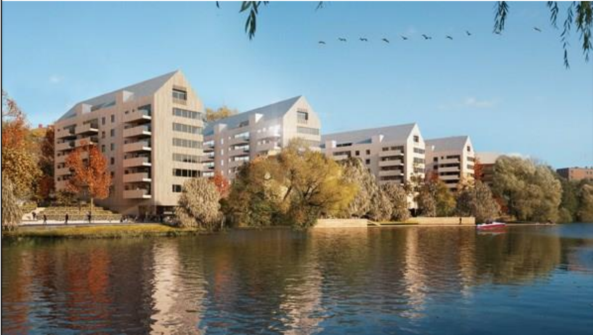
Multi-family apartment buildings in eight stories built in wood in Sundbyberg, Sweden. Image from (SR, 2012)
