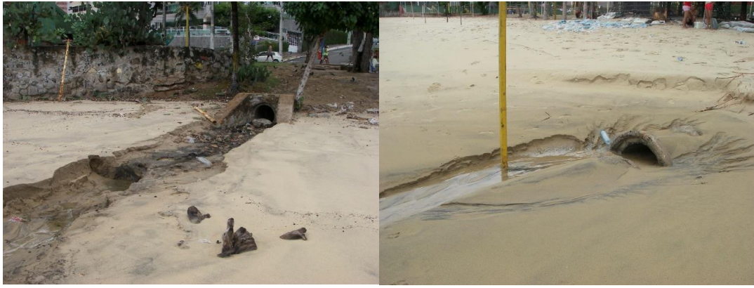
Figure 14. Storm water outlet pipes located on the adjacent beach. (Photos: Seth von Dardel, 2015)
