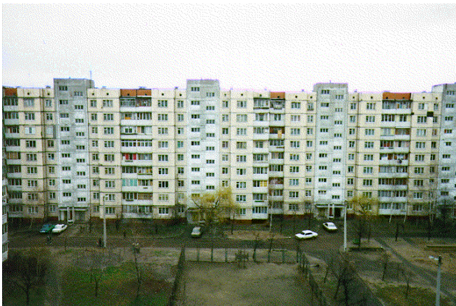
Figure 2-3 Cruiser Aurora St. building.
