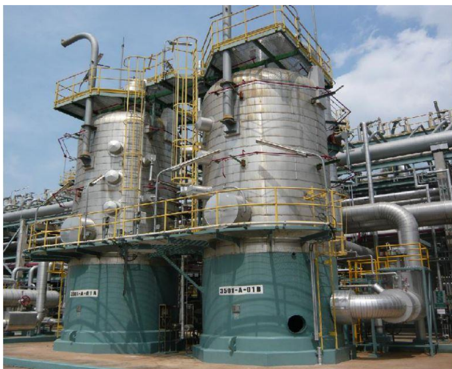
Figure 1. 7. Parallel fixed-bed reactors (MRUs) utilizing mercury sorbents at the PTT GSP-5 gas plant at Map Ta Phut in Rayong, Thailand (Eckersley, 2010).
