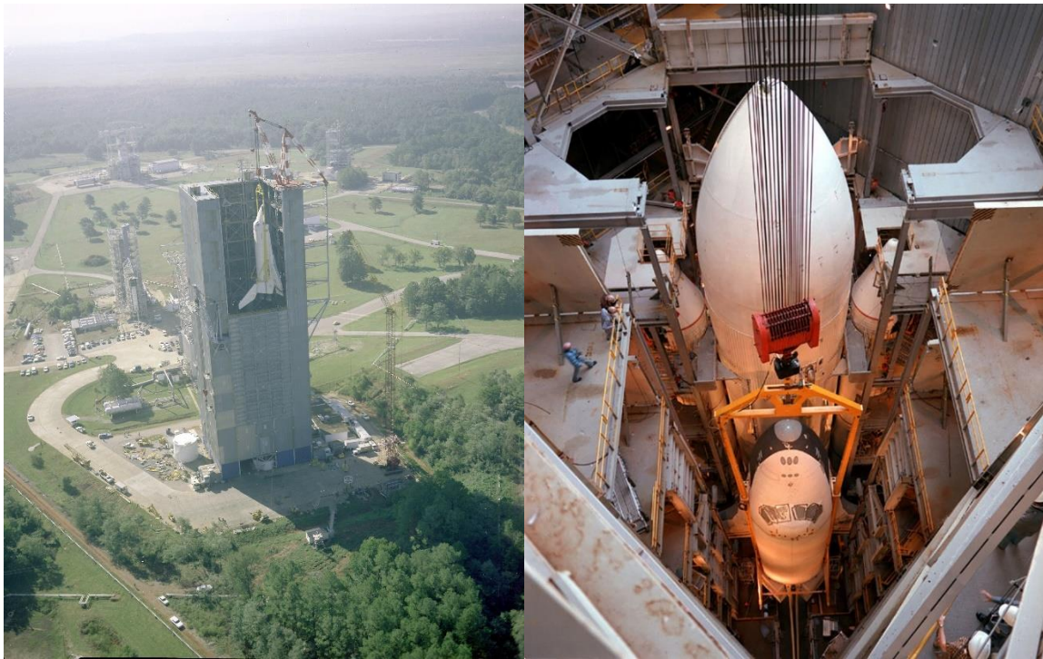
Figure 3. MSFC Space Shuttle Mated Ground Vibration Test Facility (Test Stand 4550) With Shuttle Orbiter Enterprise Being Lowered Into Place (l) And Being Integrated To The External Tank (r).
