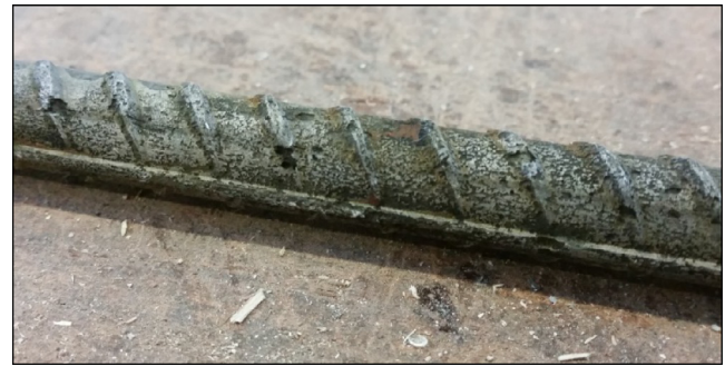
Fig. 2. Chloride induced 'pitting' corrosion of reinforcing steel.
