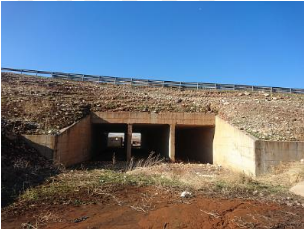
Figure 1.1 Picture of a typical reinforced concrete box culvert.
