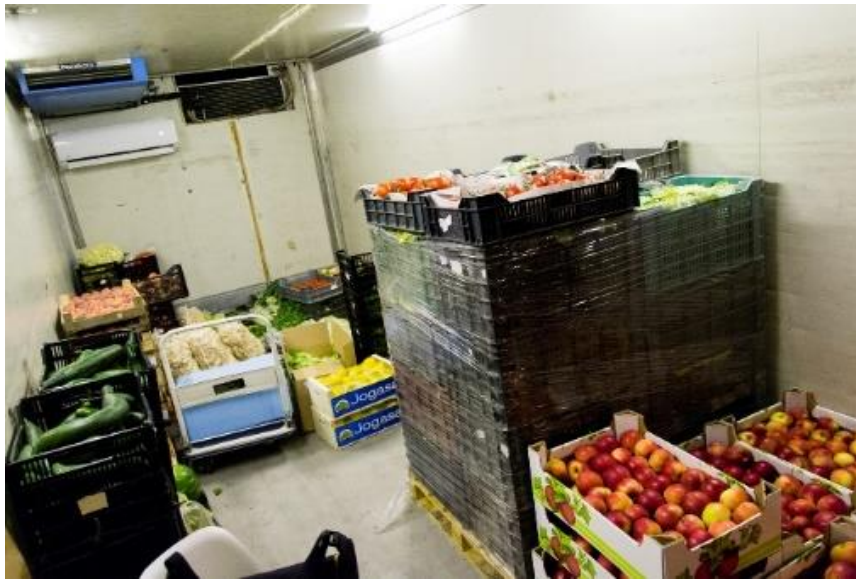
Figure 4 - Surplus food inside the tempered container, ready for redistribution
