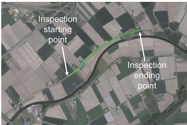
Fig. 4. Aerial view of inspected pipeline section.
