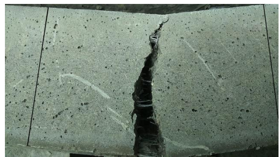
(viii) Expt. Failure crack – 26400 N
