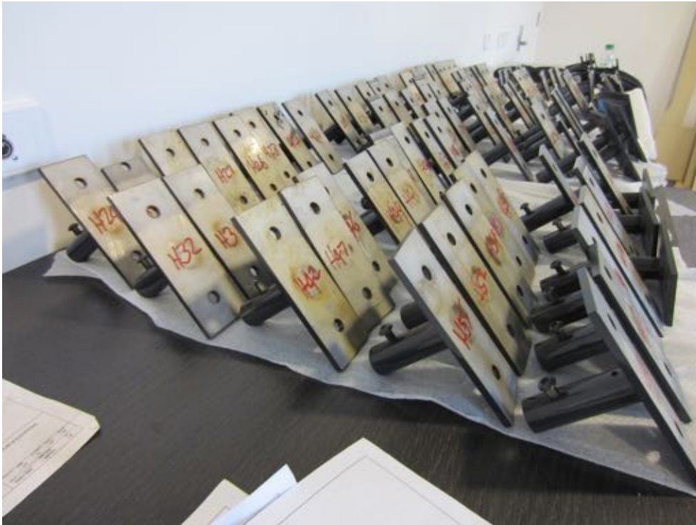
Figure 2.51 Numbered brackets in preparation for wall mounting Photo – ©Simon Perry
