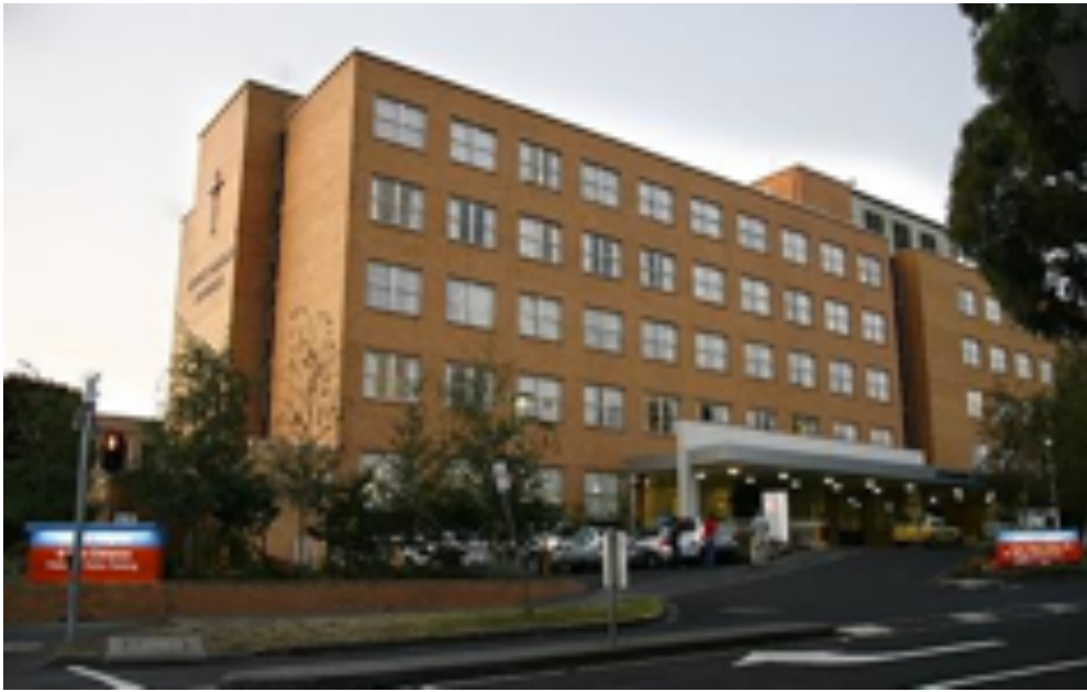
Figure 4.2 The Cabrini Hospital, Malvern, Melbourne Photo – ©Simon Perry
