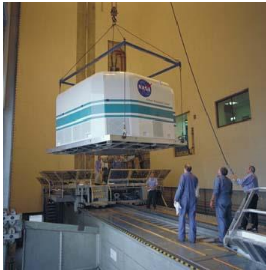
Fig. 2 Installation of I-CAB
