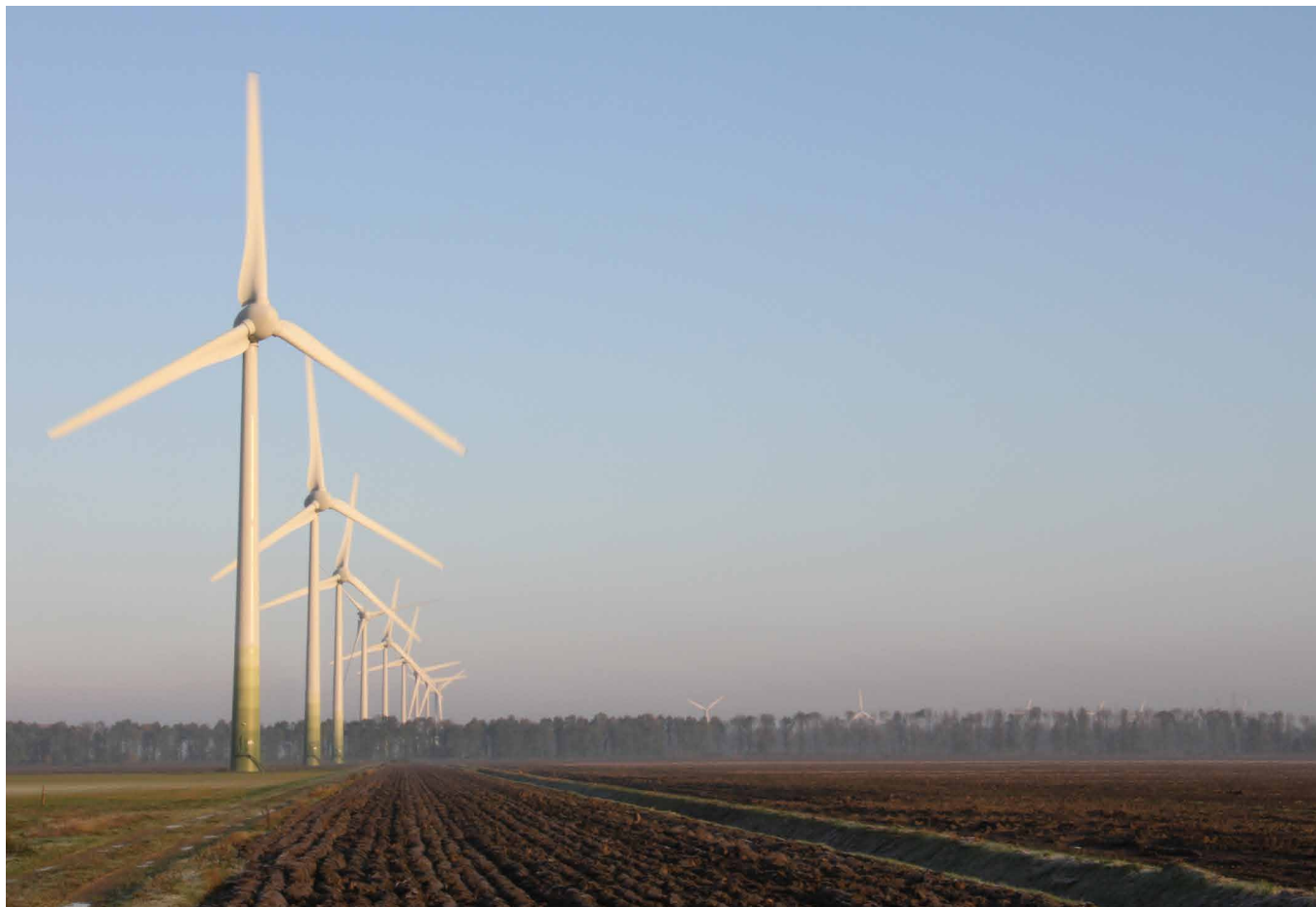
Figure 1: Wind turbines of WUR in Flevoland, The Netherlands (photographer: Andrea Terbijhe).
