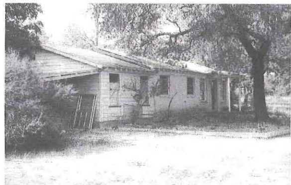
Figure 25. View to the southwest of Historic Resource No. 4, dairyman's residence.
