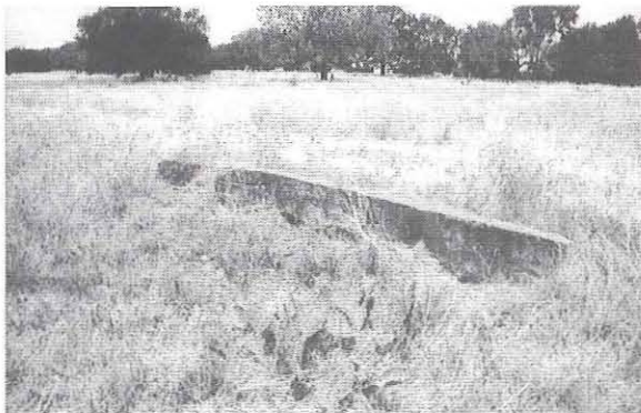
Figure 38. View to the northwest of Historic Resource No. 25a, culvert.
