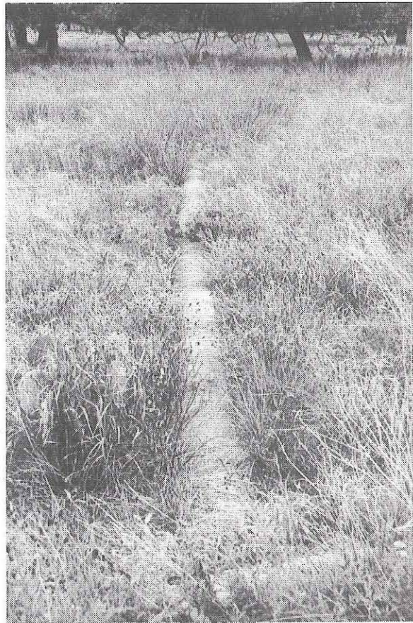
Figure 51. View to the southeast of Historic Resource No. 35, sewer pipe.
