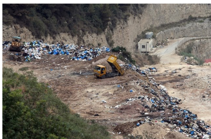
Figure 7. Solid waste piling up in Hbaline dump which led to a landslide. Source: Authors (2018).
