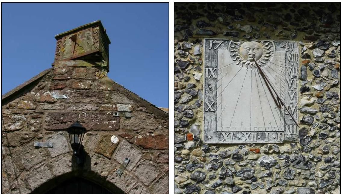
**Figure 1.6** – Sundials compensating for the poor east-west alignment of the church - “canted-out” at St Mary’s, Gilcrux, Cumbria (church @ 64°) (left), “offset gnomon” at St John’s, Ickham, Kent (church @ 108°) (right)
