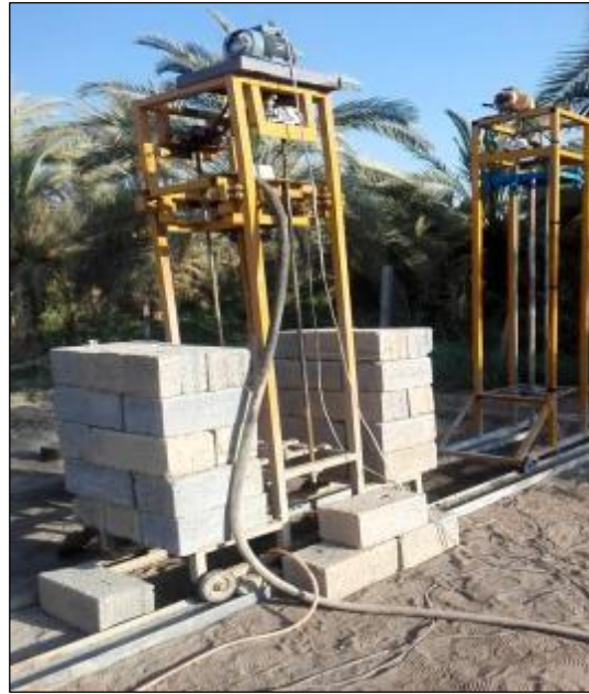
Figure 3. Jet grouting machine
