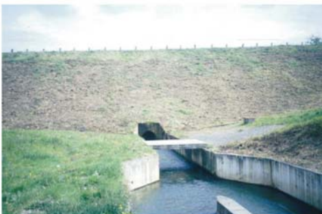
Photo 5: Outlet from the bottom conduit for the monk at Pouge Pond (commune of Saint-Auvent) seen from the emissary (photo L. Touchart, 1998)
