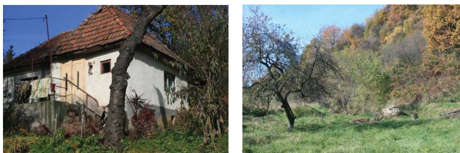
Figure 5. Landslide from Plaiului street
