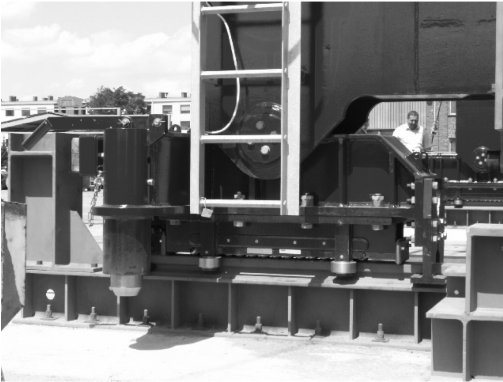
Fig. 6. Connecting the gantry crane to the deck Rys. 6. Posadowienie suwnicy BOP
