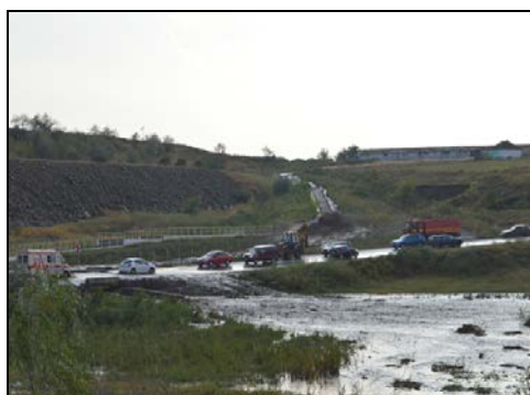
Fig. 4. Overflow over the bridge on DN 22
