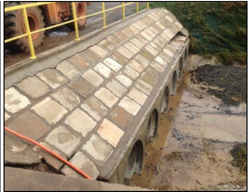
Fig. 7. Bridge over concrete tubing
